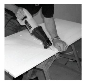
Continue to lay the master panels. When cutting the master panels, mark the plate and saw it with EPS side up. You can use any saw with a fine-toothed metal blade. After cutting the panel, remove any burrs. When cutting the last master panel in the first row, use the rest of the panel to start the next row. This will provide staggered joints for the field panels.
