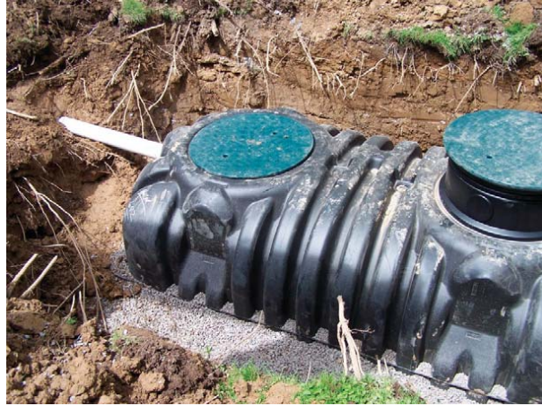
Photo 4.1.9-Uniform level distribution of material
