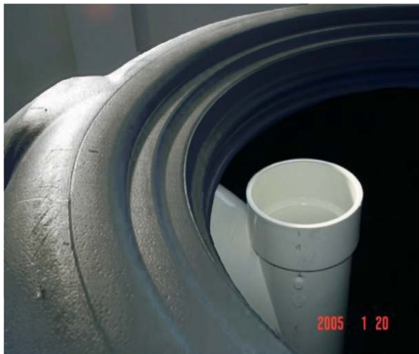
Photo 4.1.16-Pipe located inside the edge of the manway
