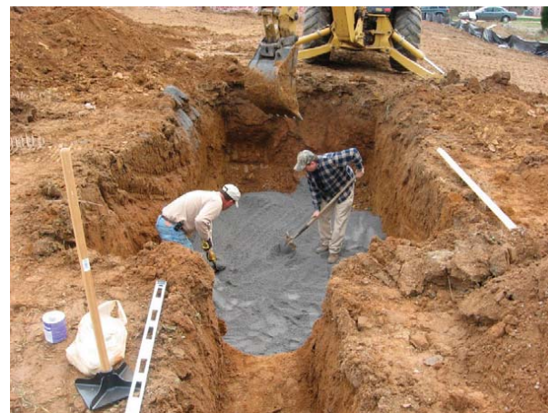
Photo 4.1.3-Bedding being spread and compacted
