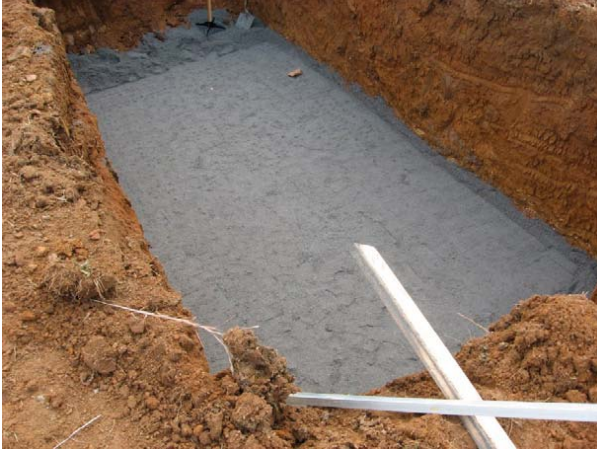
Photo 4.1.4-Bedding material prepared for setting the tank
