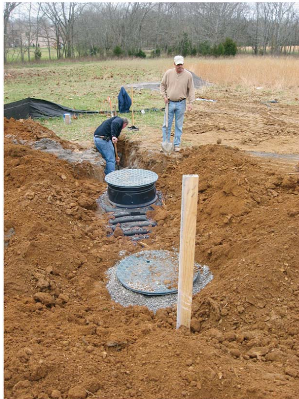
Photo 4.1.12-Example of complete backfill
