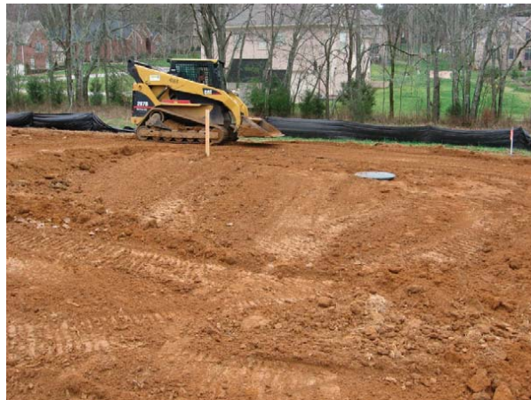
Photo 4.1.14-Example of final grading
